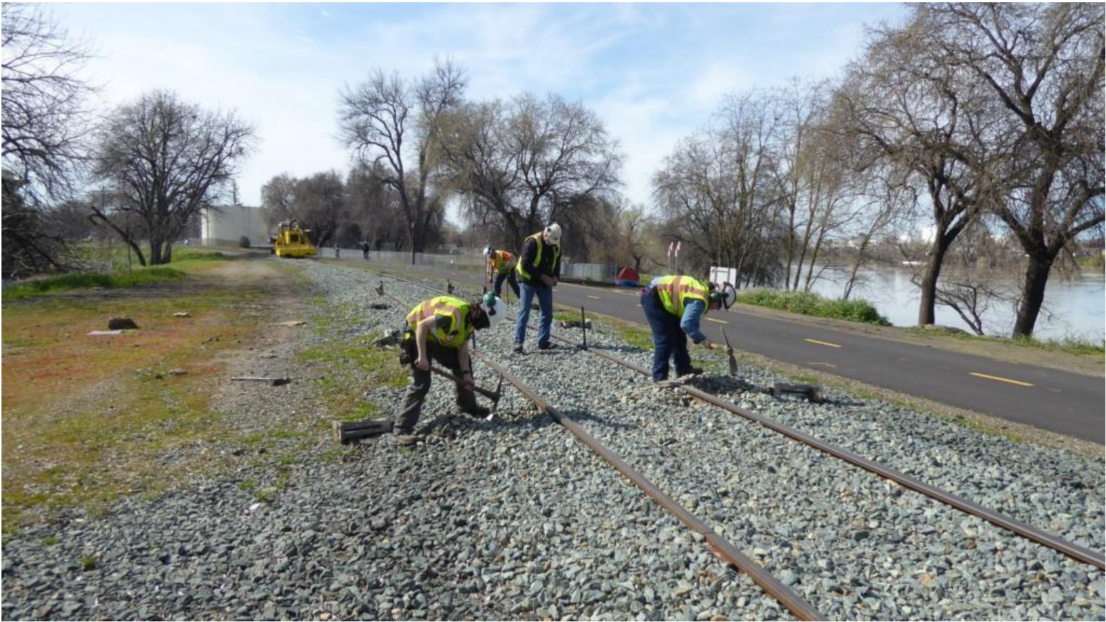
Matt and Heather dig pockets under the base of the rail for jacks while Alan sets up the spot-board
