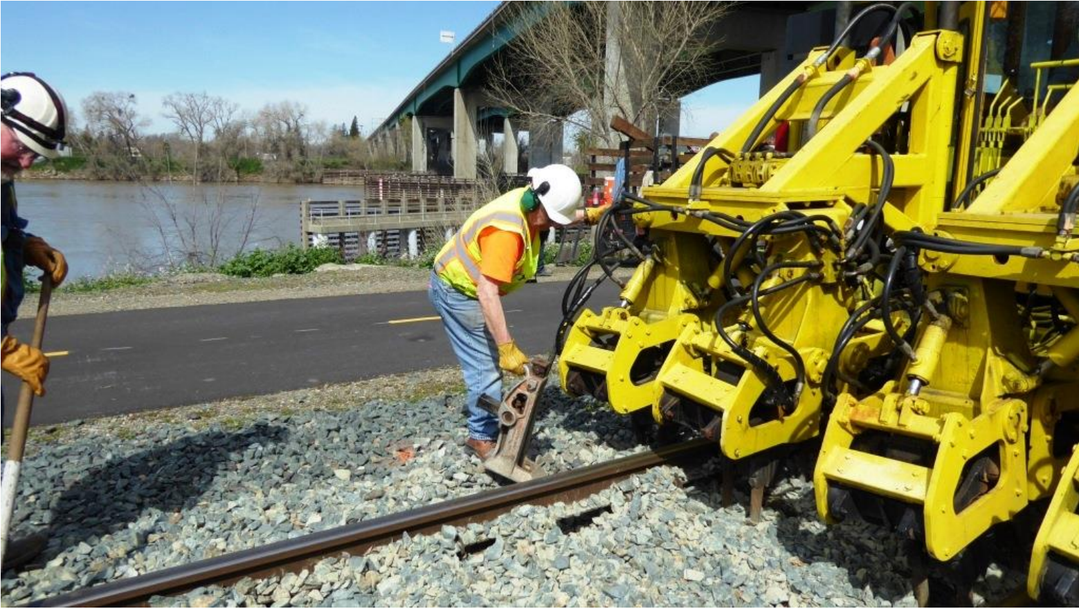
Mike W. pulls a track-jack as the tamper approaches
