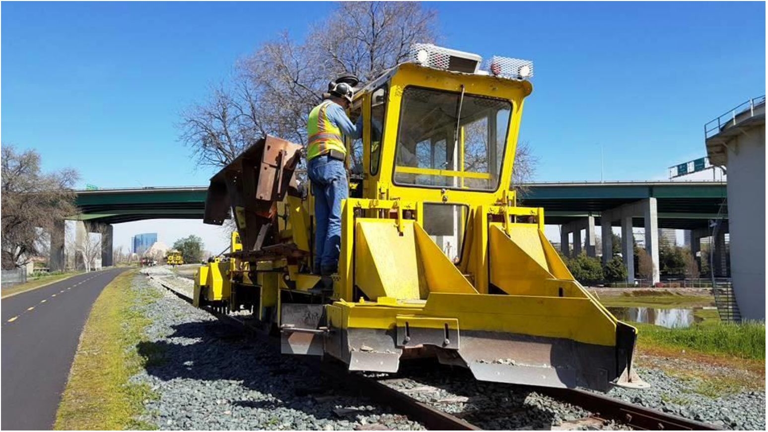
Alan takes a ride as the ballast regulator plows the rock evenly between the rails
