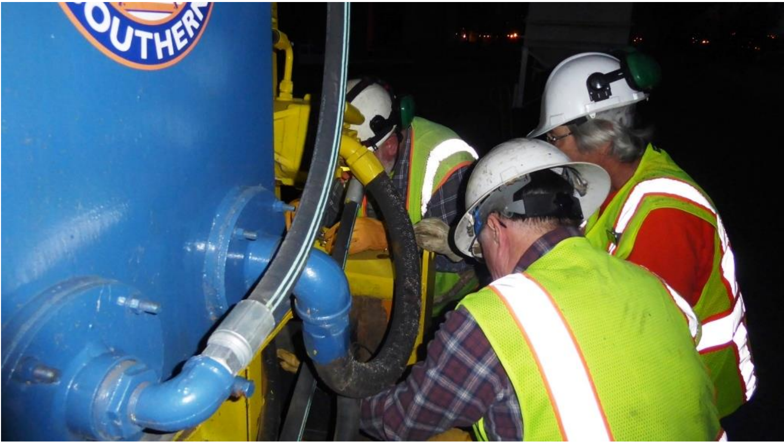
Mike H., Ed, and Frank install a new battery in the tie-crane
