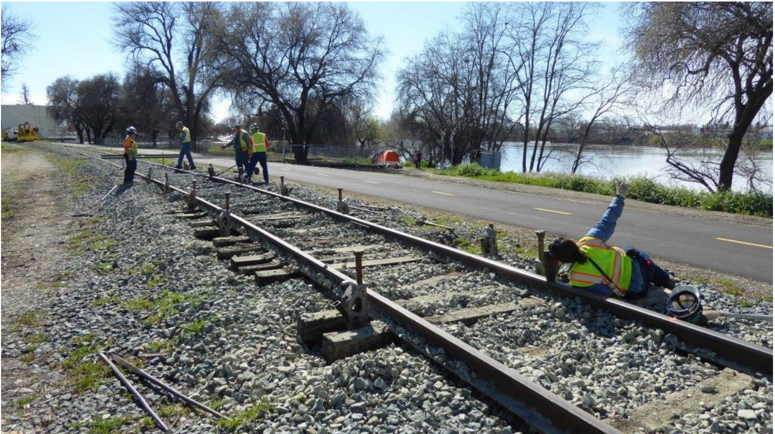
Heather measures the run-off and signals to Ed and Frank on the track-jack
