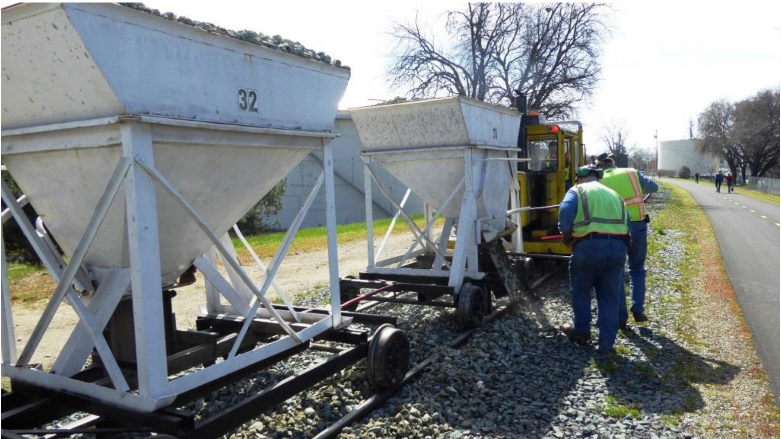
Frank and Alan drop ballast rock from the side-dump car
