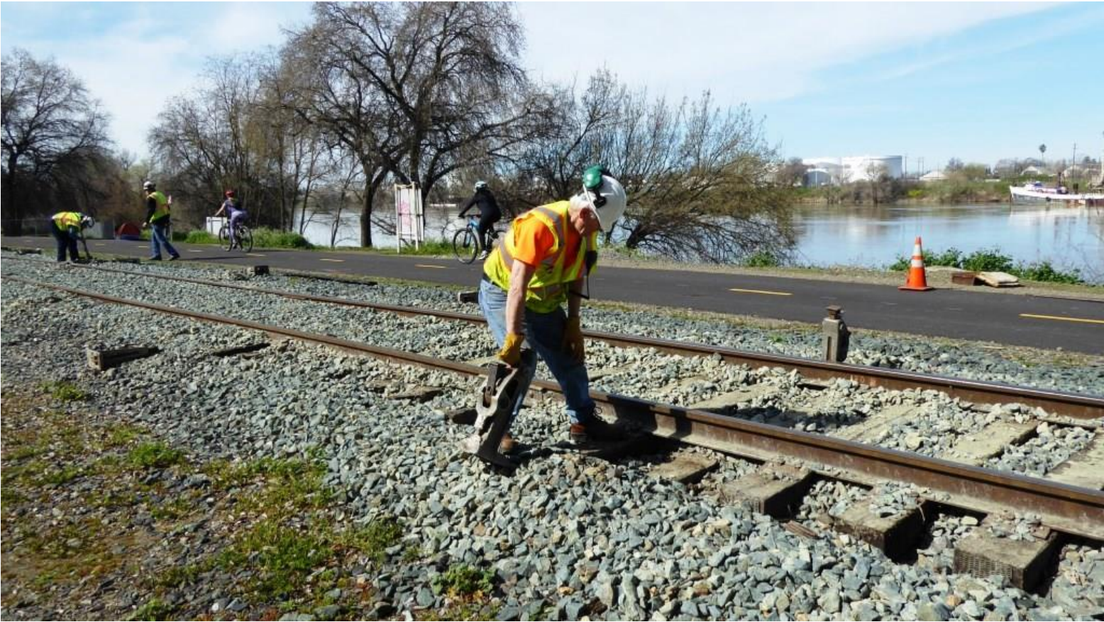
Mike W. gets a track-jack ready to place under the base of the rail
