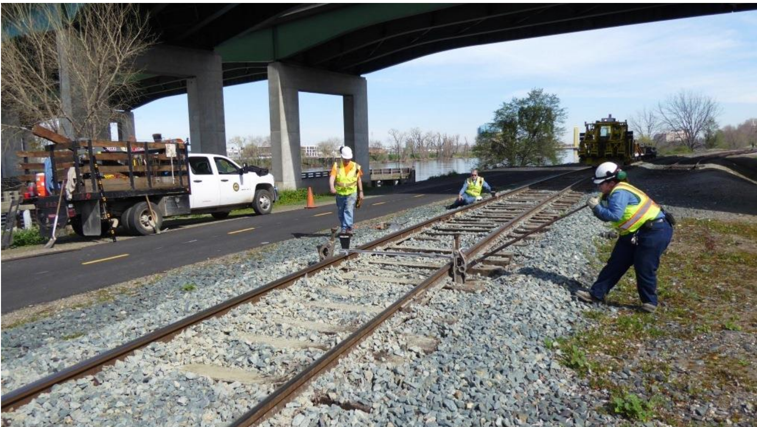
Alan behind the "hound" as Heather jacks the east rail level with the west
