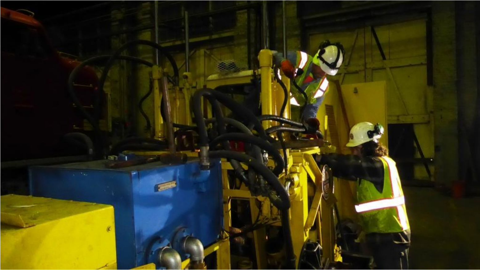
Joe and Matt work on the re-plumbing of the tie-shear
