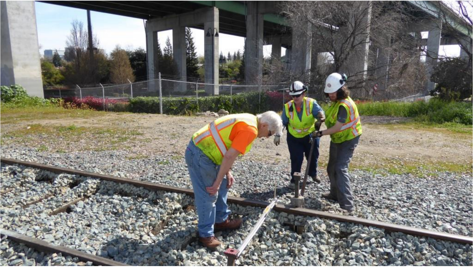
Mike W. checks the track-level as heather and Matt raise the east rail
